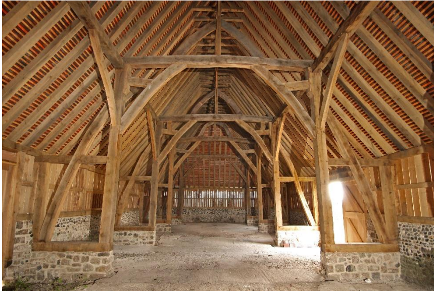
Pl 12: Interior of restored northern bays of barn, looking north in 2019.
