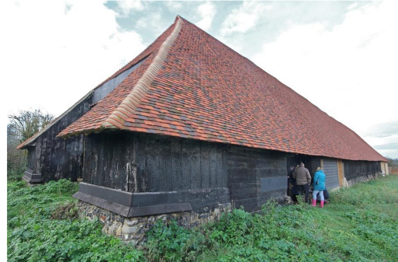
Pl 10: View of restored barn, looking north-west in 2019.
