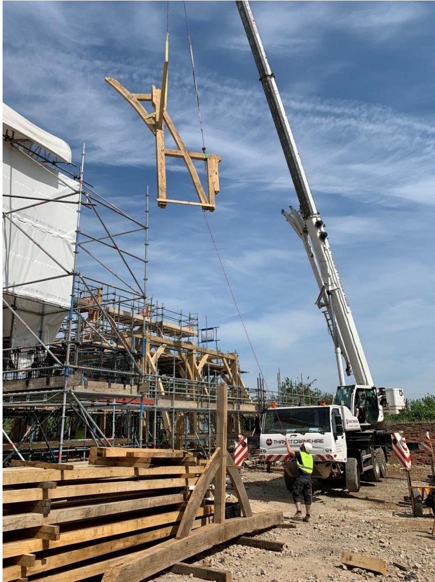
Pl 9: New oak framing being hoisted into position at north end of barn during restoration in 2019.
