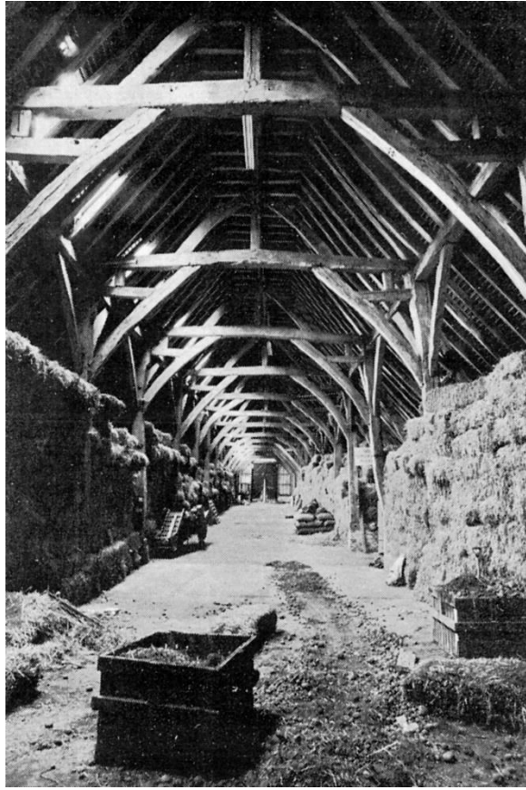
Pl 4: 1970-80s view of barn interior, showing it in use for storing crops.
