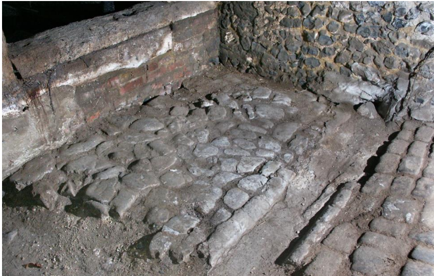
Pl 7: Remnants of Kentish Ragstone paving and open drain in south aisle of barn.
