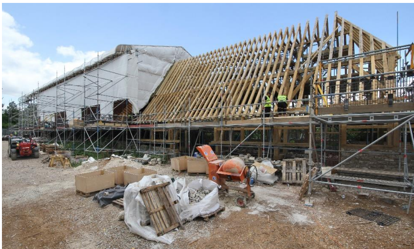
Pl 8: North end of barn, showing bays 1-4 during reconstruction in 2019.
