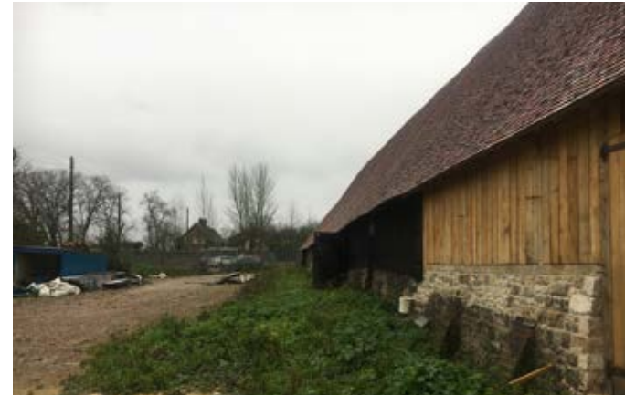
Figure 11 | External view of barn
