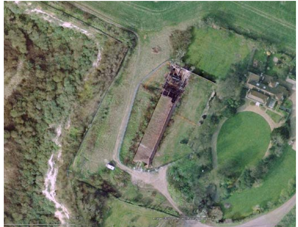
Figure 23 | Aerial photo post the fire to the northern bays (2003 - google maps)
