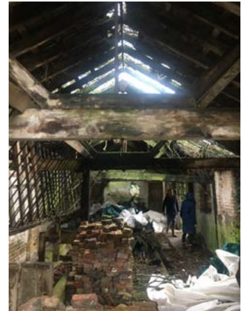
Figure 6 | Internal view of cowshed
