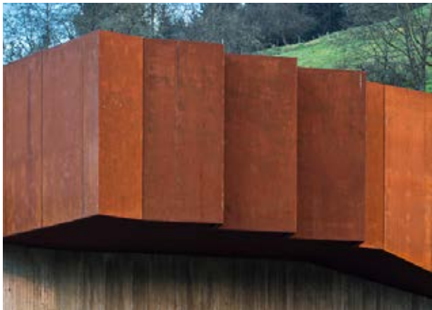
Figure 54 Corten Steel cladding
