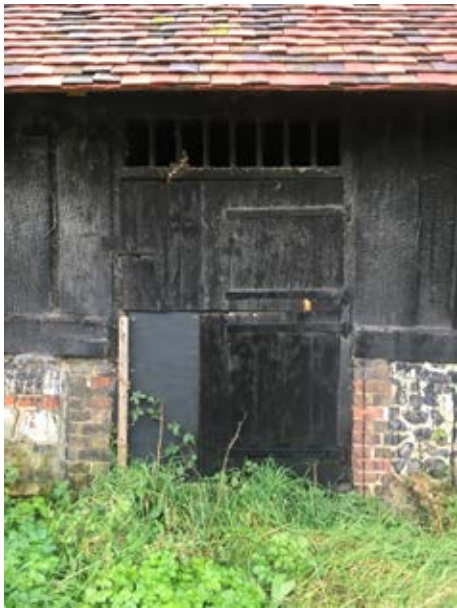
Figure 7 | Historic End of the barn with black tar finish
