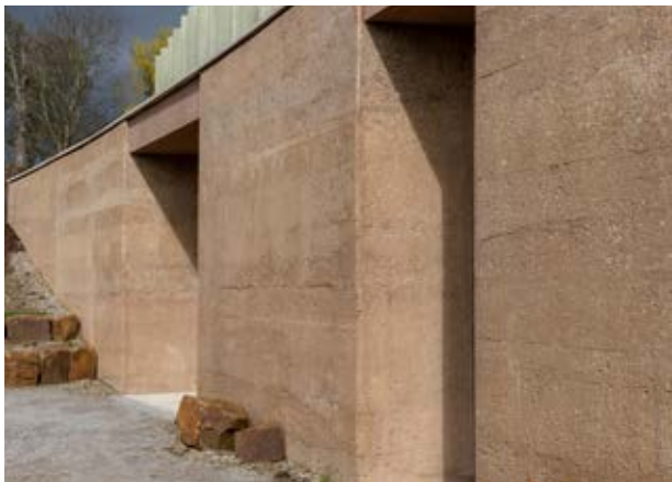
Figure 55 Rammed Earth Finish layered pigmented concrete
