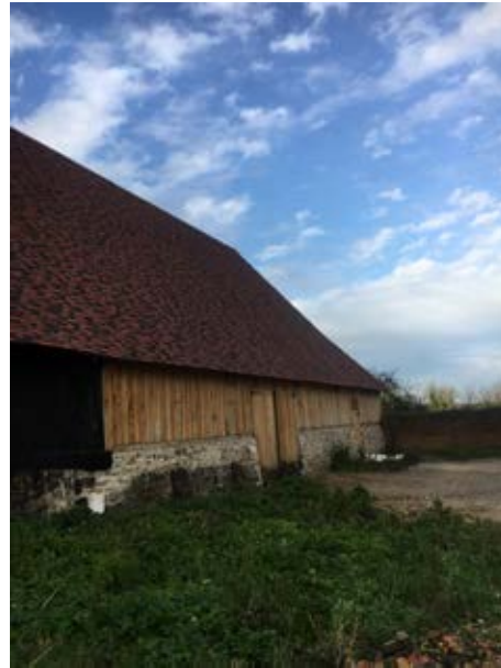
Figure 8 | Re-built end of the barn without final tar finish
