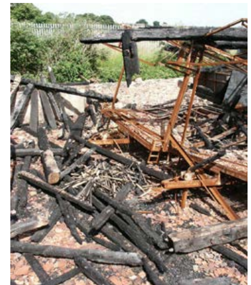
Figure 25 | Aerial Photograph and images of fire damaged barn
