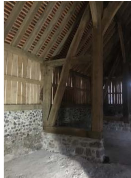
Figure 9 | Internal view of re-built end of the barn
