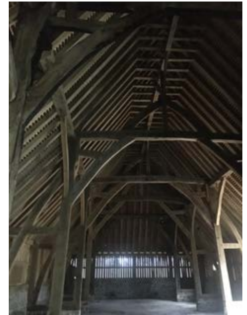
Figure 10 | Internal view of re-built end of the barn
